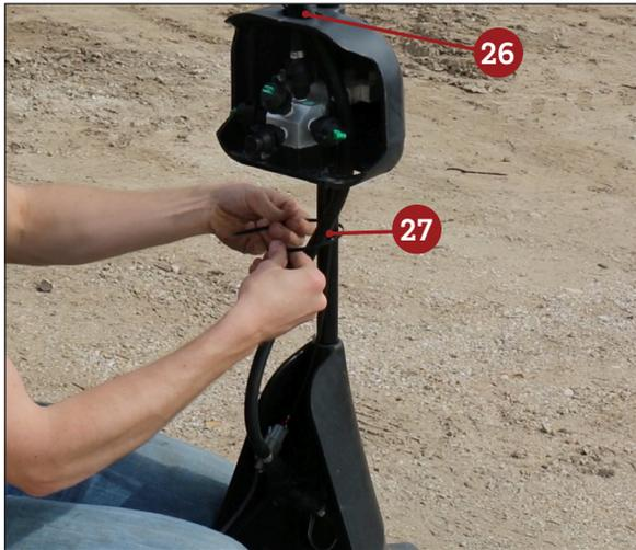
Reinstall the 360 Y-DROP hose, and if applicable, the 360 UNDERCOVER hose **26** by routing them from the OEM boom down through the 360 UNDERCOVER unit to the Y-DROP base unit.
