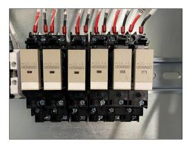
Starting from the left the relays are Output 1, Output 2, Output 3, Output 4, Output 5, Output 6.
