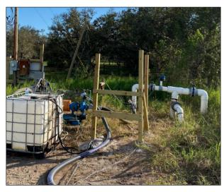
Posts: Three 4"x4" posts positioned 3ft apart and secured together with 2"x6" and 2"x 4".
