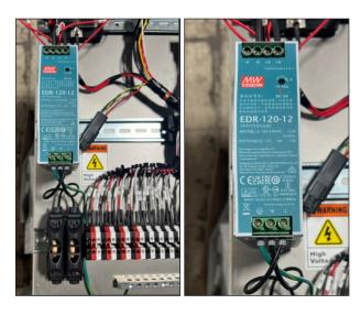
The base station box comes standard with a 120 V AC single phase power supply.
